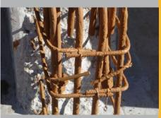
Major repairs required us to remove the existing plinth to expose the reinforcing which was then cleaned and primed in preparation for new plinths to be poured.
