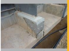
Where repairs were minor, injection holes were drilled into the cracks, ports installed and resin injected into each hole; once cured the ports were removed.
