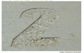
Sand-blasted concrete can result in a bold pattern
