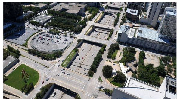
Figure 4: Klyde Warren Park before—Dallas, TX
