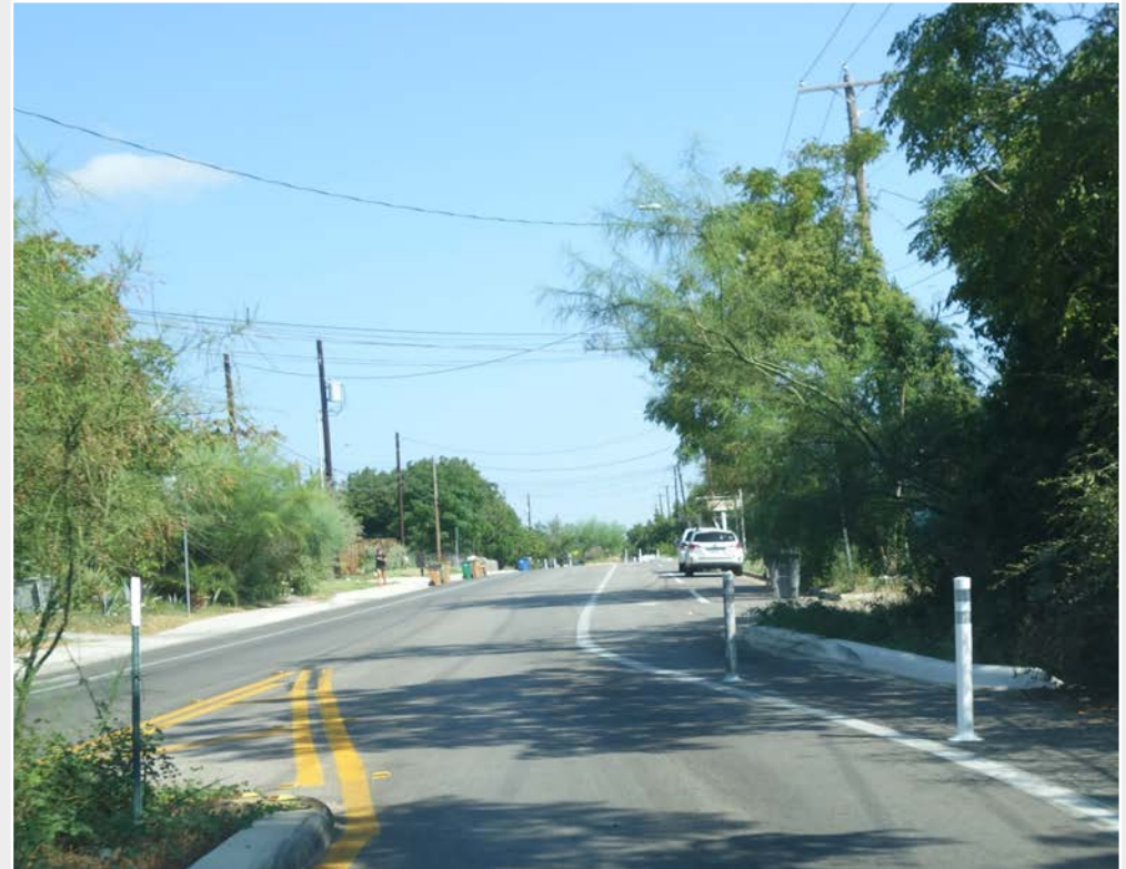
NPP street safety project on E.M. Franklin Avenue.
