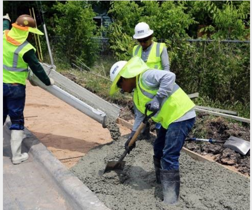
Sidewalk crew at work.
