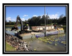
Use of silt curtains when turbidity is an issue. Spuds hold the barge in place for extra stability and precision. This work in Maroochydore - excavating before rock armouring.
