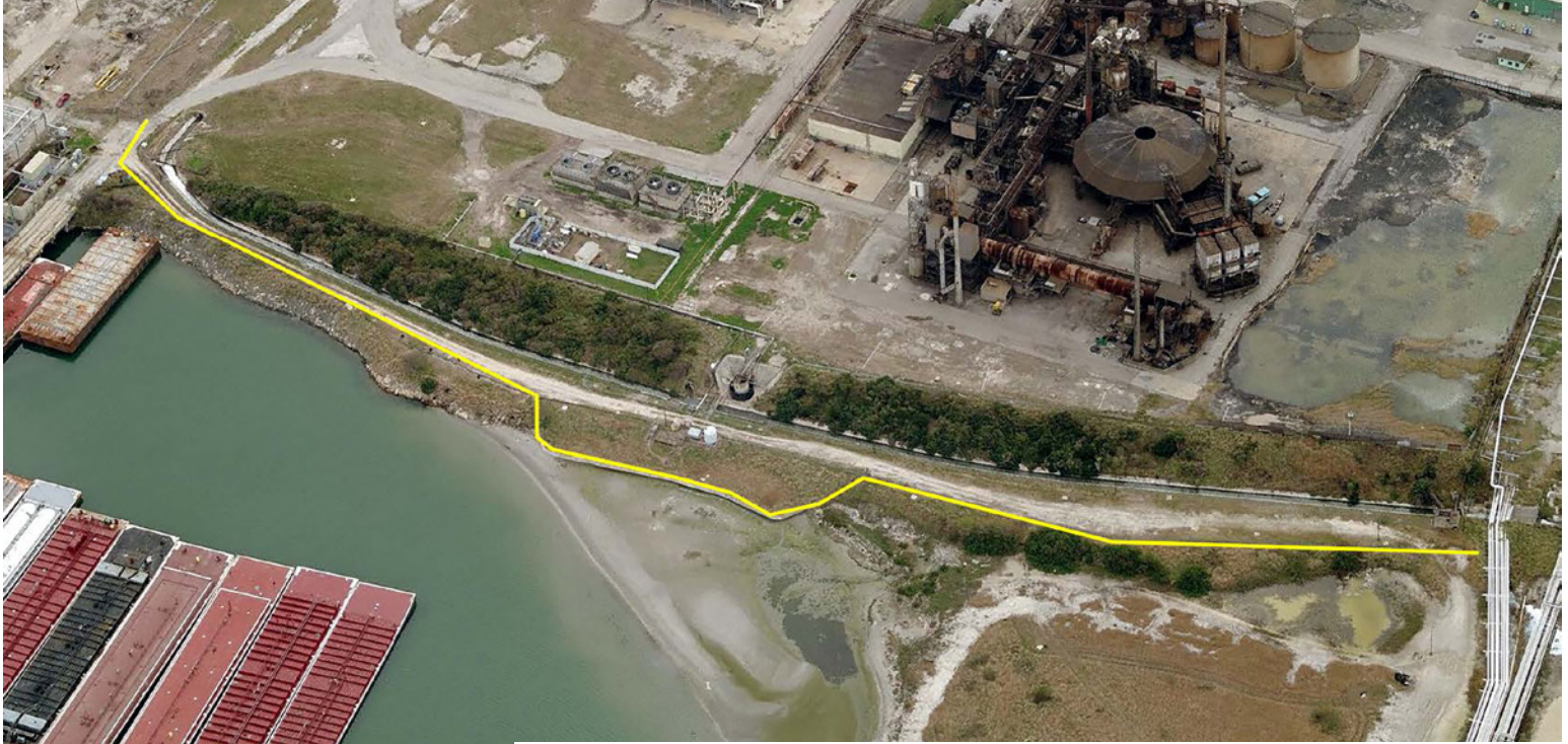
Elementis Subsurface Barrier Wall | El Paso, TX | November 2009
