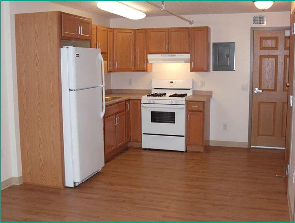
Figure 4. Orness Plaza, a public housing complex in Mankato, Minnesota, was renovated to meet Enterprise Green Communities criteria and LEED® Silver certification. HVAC improvements included range hoods that vent outdoors. Photo courtesy Blumenthals/Architecture.
