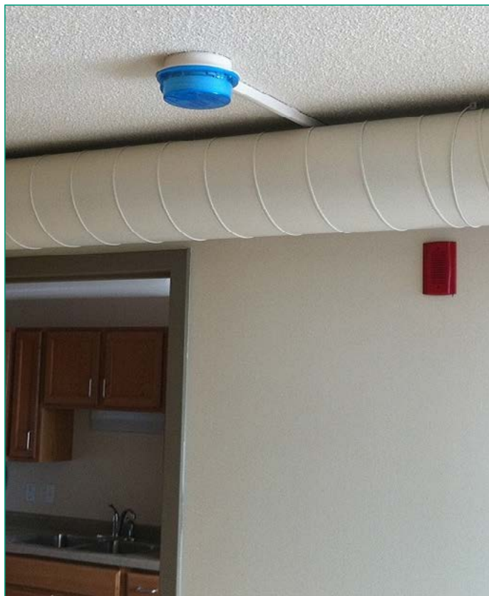
Figure 2. Orness Plaza, a public housing complex in Mankato, Minnesota. Between 2010 and 2012, the property was renovated to meet Enterprise Green Communities criteria and LEED® Silver certification. The addition of a carbon monoxide detector can have profound benefits in a living space. Projects involving simple enhancements, such as air sealing, addition of insulation, or heating upgrades were also evaluated for health benefits. Photo courtesy the National Center for Healthy Housing.
