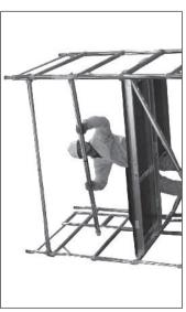
From the sitting position through the trapdoor (3T), fit four handrail braces to vertical member of frames. 17
