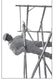
Fit four handrail braces, two on outside and two on mid rung of frame as shown, on lower levels these may not be required.
