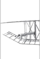
Continue erecting tower to final tower height repeating the 3T process as illustrated. Always ensure that there is side protection to prevent falls. Maximum vertical distance between platforms must not exceed 4m. 女
