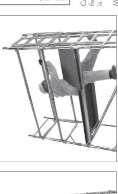
Fit trapdoor platform on appropriate rung. tower illustration for guide.
