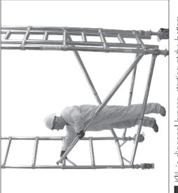
Klik in diagonal braces, starting at the bottom rung. Single width towers have 2 braces at the base and singular thereafter. Braces should be in a continuous pattern from rung to rung except when interrupted by an intermediate platform.
