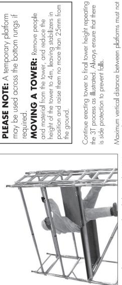
From the sitting position through the trapdoor (3T) fit four handrail and mid rail braces to the vertical members.
