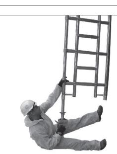
Insert two adjustable legs and castors into frame.
