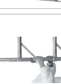
After adding frames engage interlock clips
