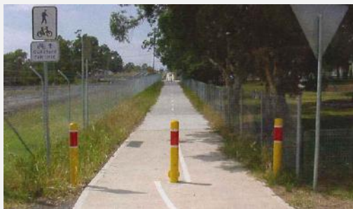
Steel Bollard: Access restriction, containment unknown, impact behaviour unknown.
