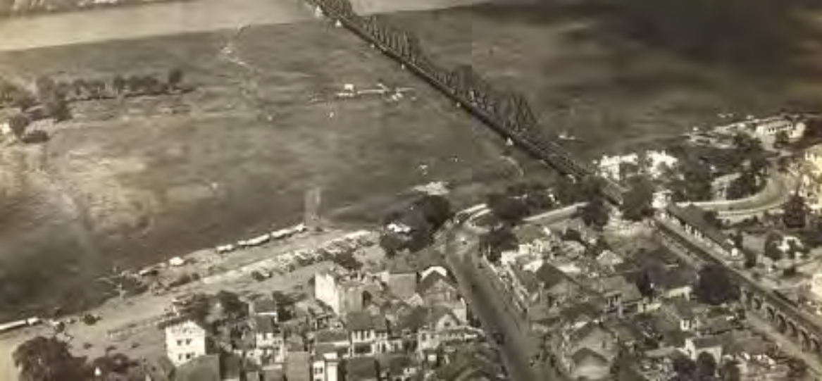
From Hang Co Railway station to Long Bien bridge (beneath is the mural arches in Phung Hung street)
