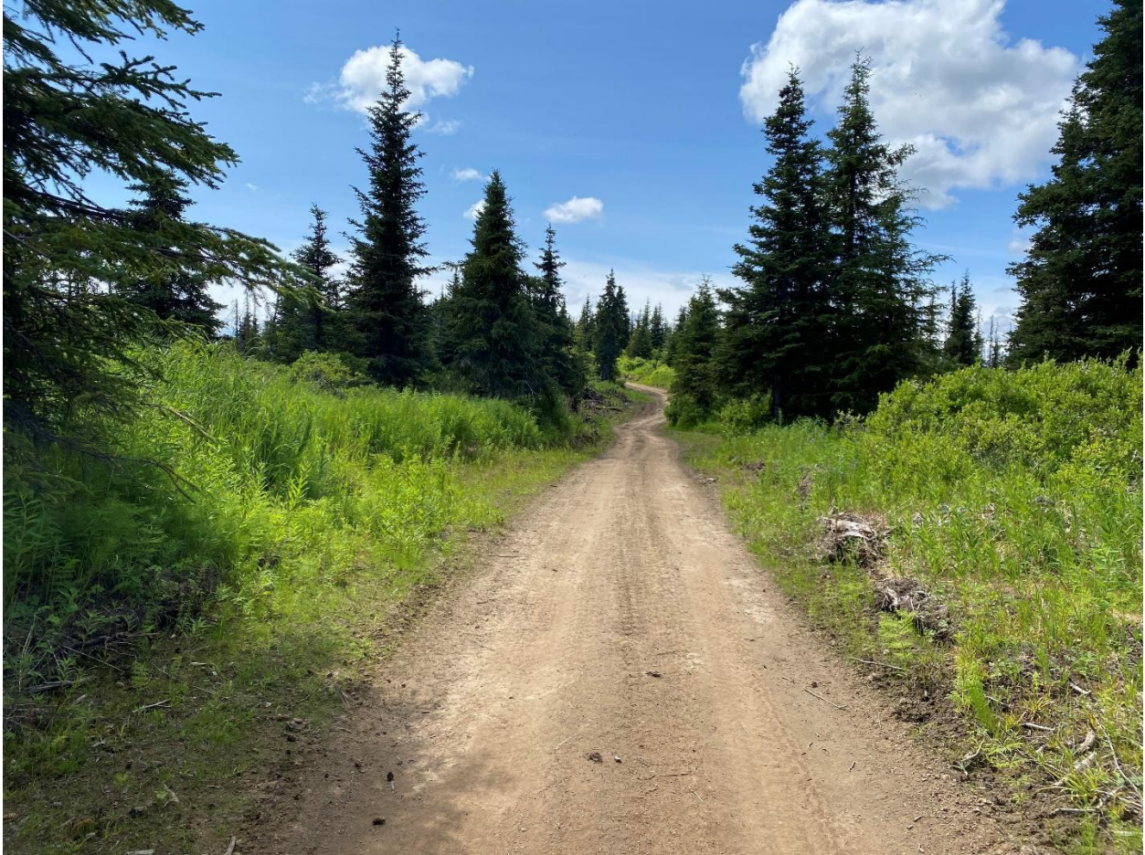
Photo 3: The portion of the Boardwalk Trail between the parking lot and the Moose Creek. This section was partly rehabilitated in 2021.
