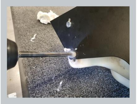
If you are using the top set of holes for your installation, the tank's 4<sup>th</sup> mounting hole will line up with hole 4 in the bracket, so you can skip this step. If you are using the bottom set, you will need to drill a slot in the tank matching the one in the bracket (hole 4).
