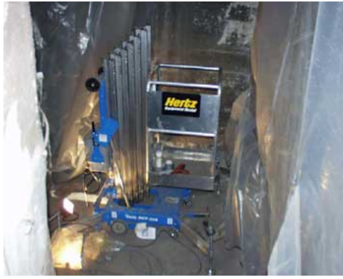
Attachment 2. Genie 30' Single Person Electric Platform Lift being used on site.
