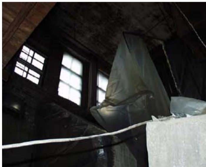
Attachment 4. Plastic sheeting that fell during accident.
