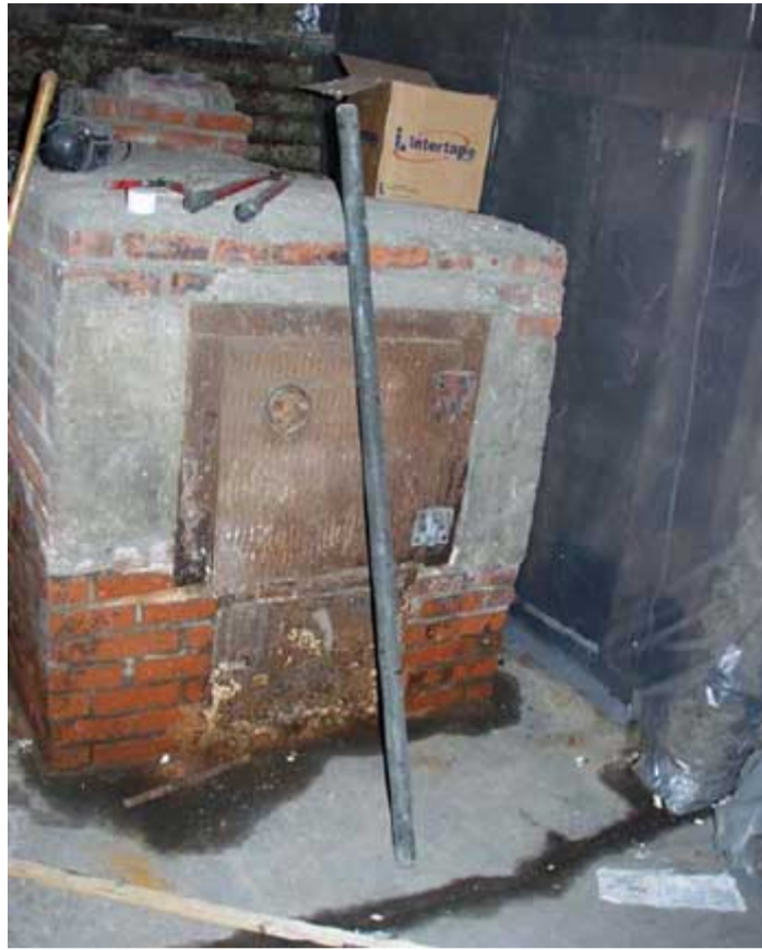
Attachment 5. Metal pipe being used to brace boards/sheeting.
