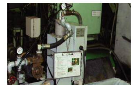
Collecting non-ferrous sludge such like abrasive grains after magnetic filter
