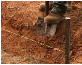
1. Stake out / remove sod
