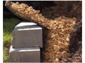
5. Add drainage aggregate
