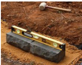
4. Lay and level blocks
