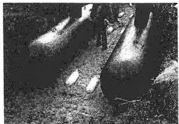
EXHIBIT 6.17 Installation of Two Underground Tanks, Showing Placement of Anodes. (Courtesy of H&H Gas)
