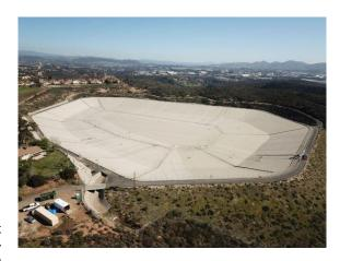
reservoir covers 17 acres and has a maximum depth of 60 ft. Interior side slopes range from 2H:1V to 4.5H:1V. The reservoir geometry is complex, consisting of eight curves and eight tangent sections.
