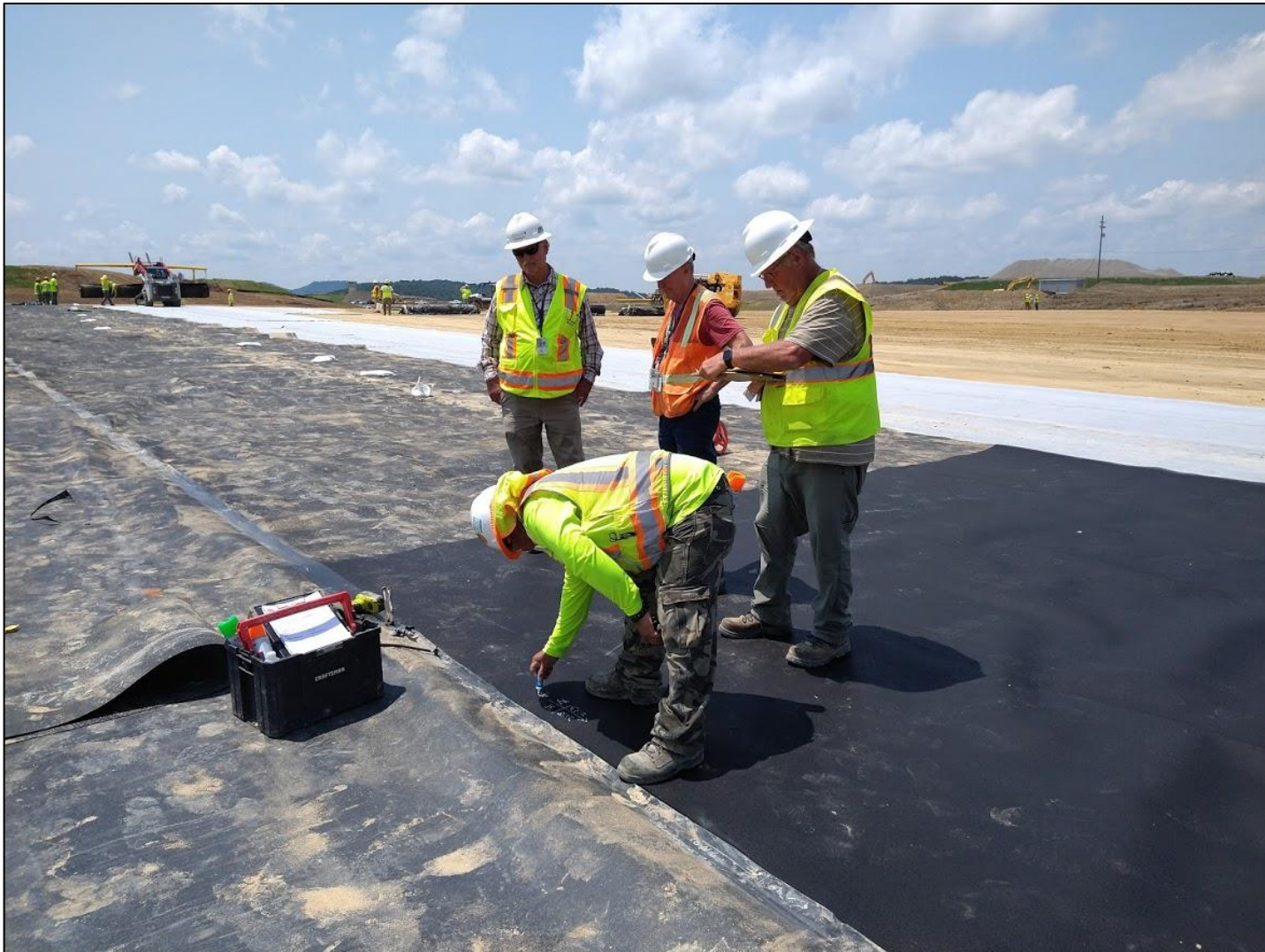
Typical Quality Control and Quality Assurance Air Channel Testing
