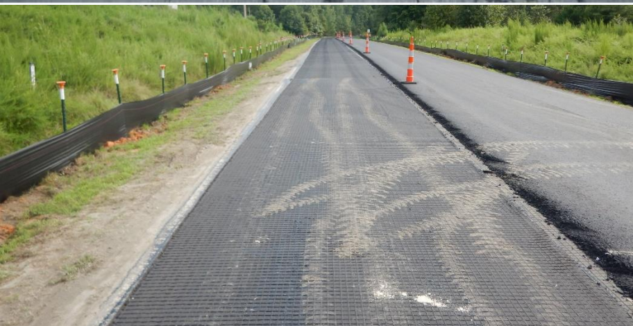
Pavement Condition Before Installation and Interlayer Installation
