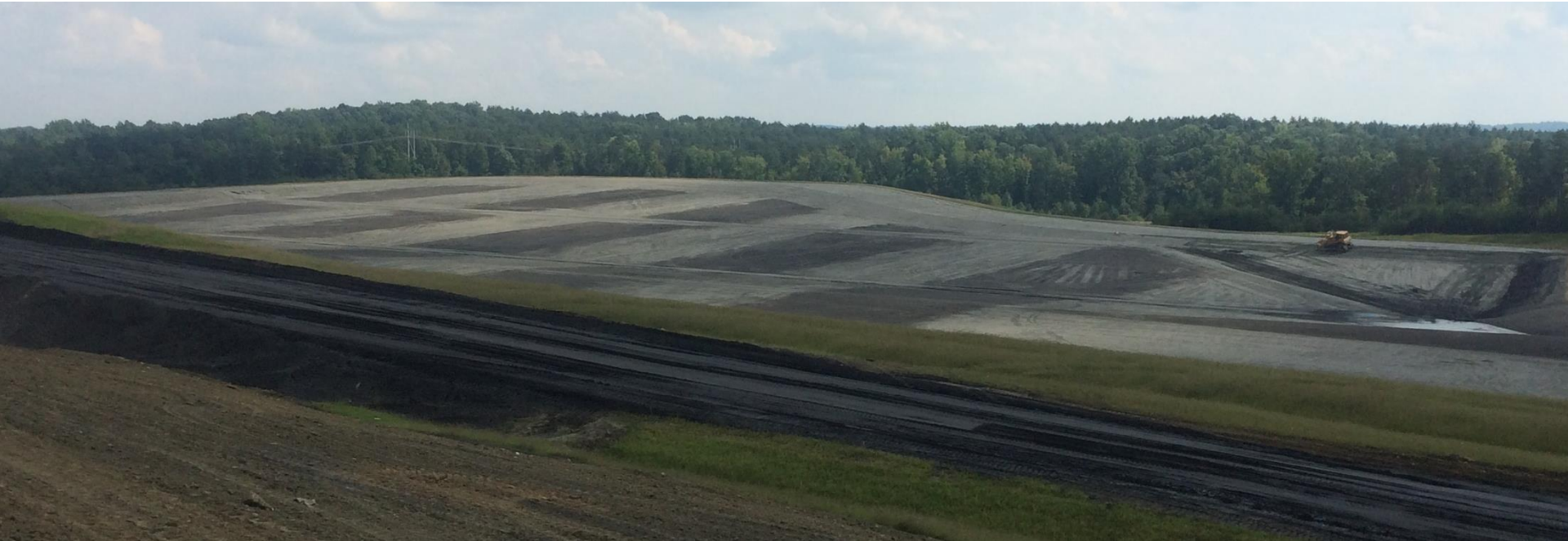
Landfill Showing Alternating Bottom Ash / Sand Protective Cover
