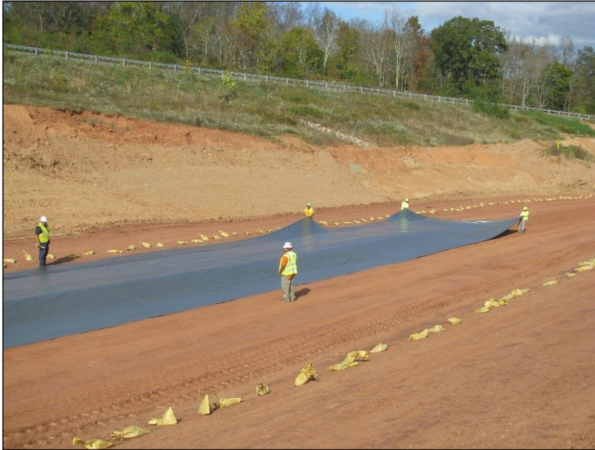
Fabricated Geomembrane Deployment
