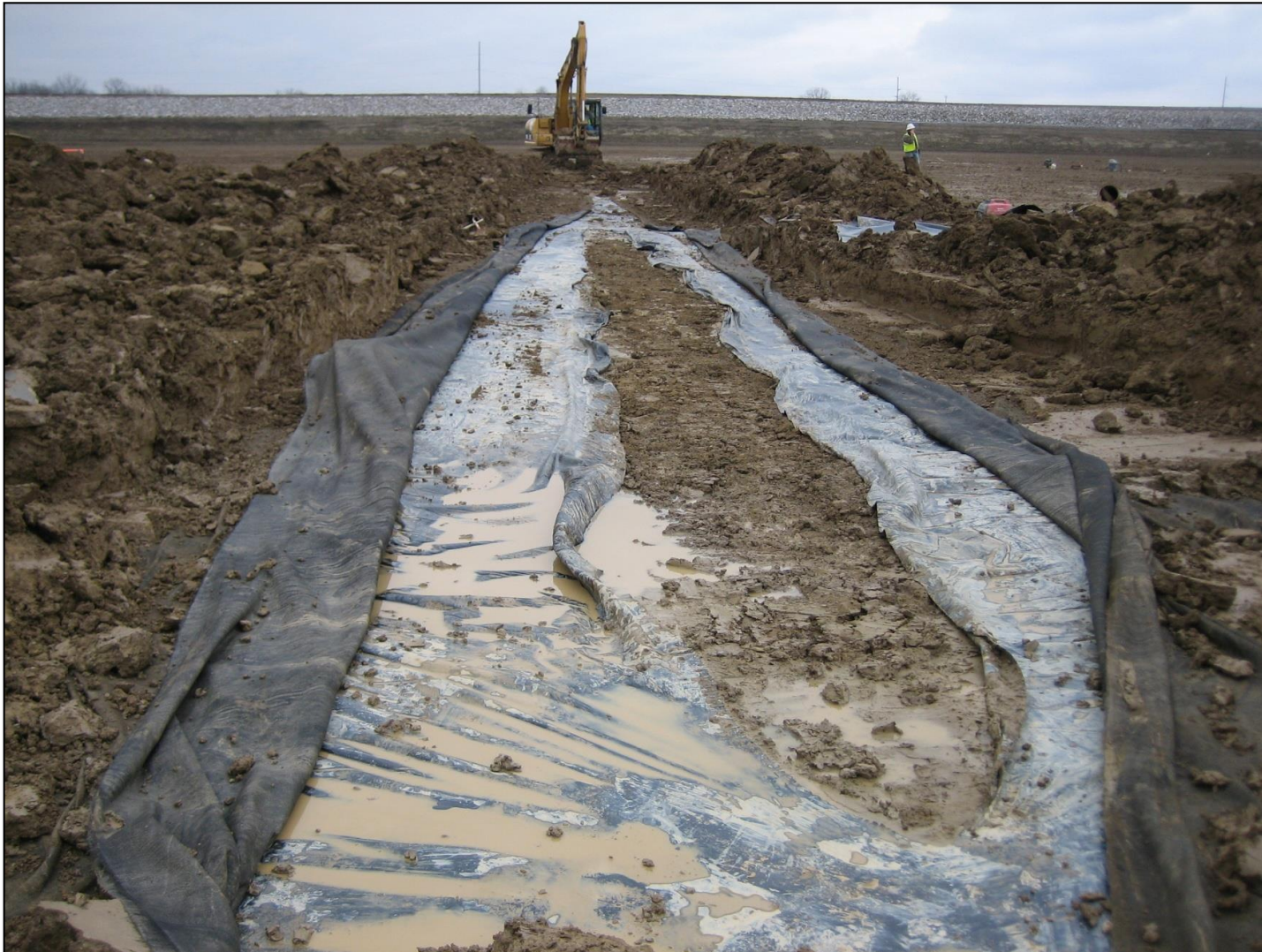
Liner Defect found from Electrical Leak Detection
