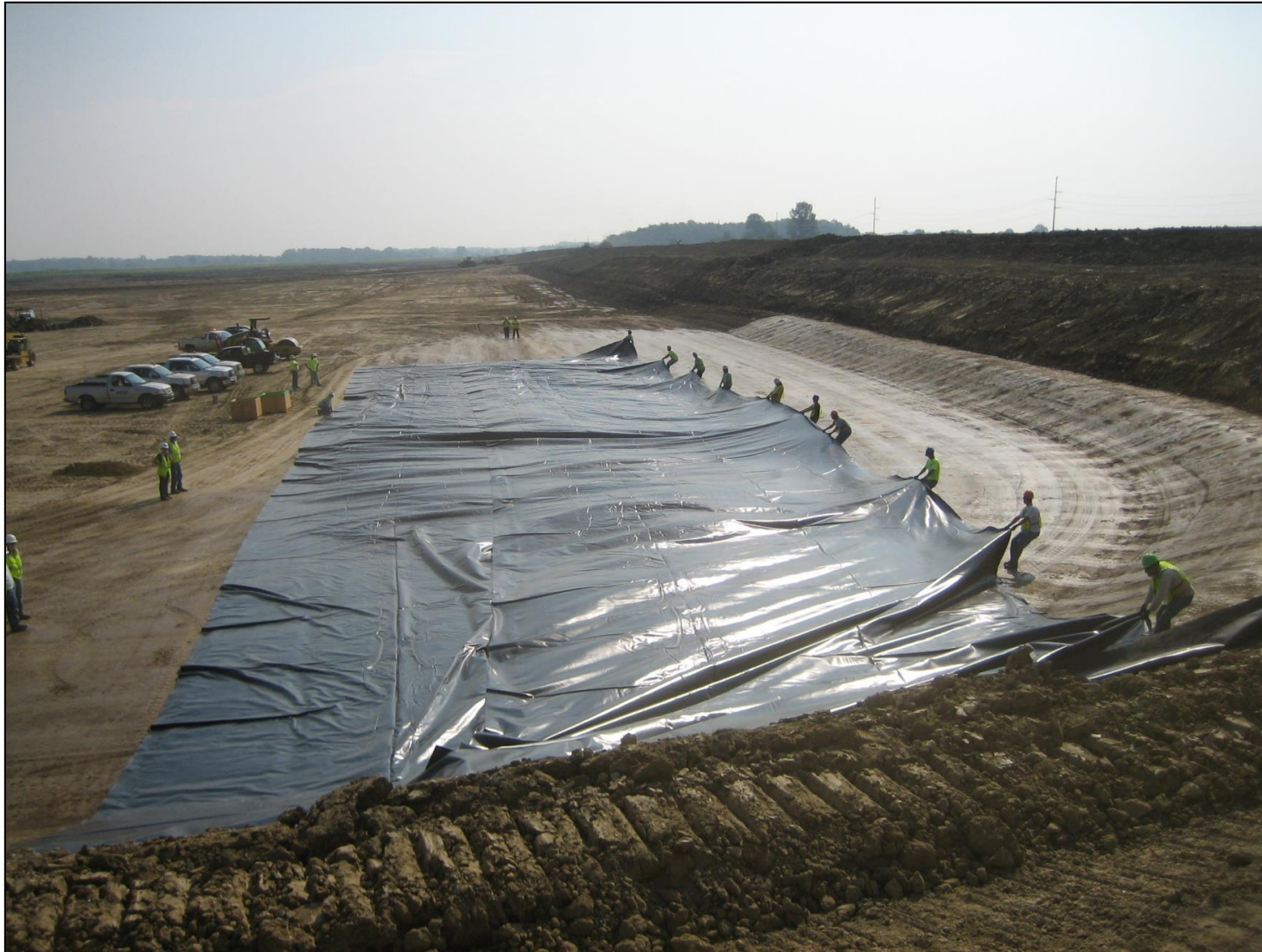
Fabricated Geomembrane Deployment – 1 Panel!
