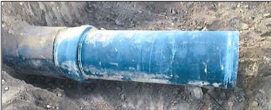
Ductile Iron Pipe Outlet
