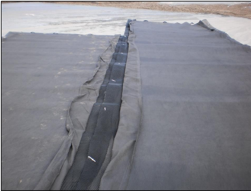
Zip tie connection of drainage net core
