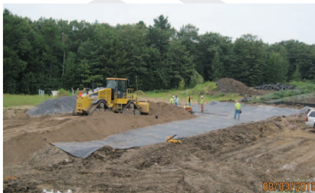
Figure 4. Test pad with HSD placing sandy structural fill on geomembrane
