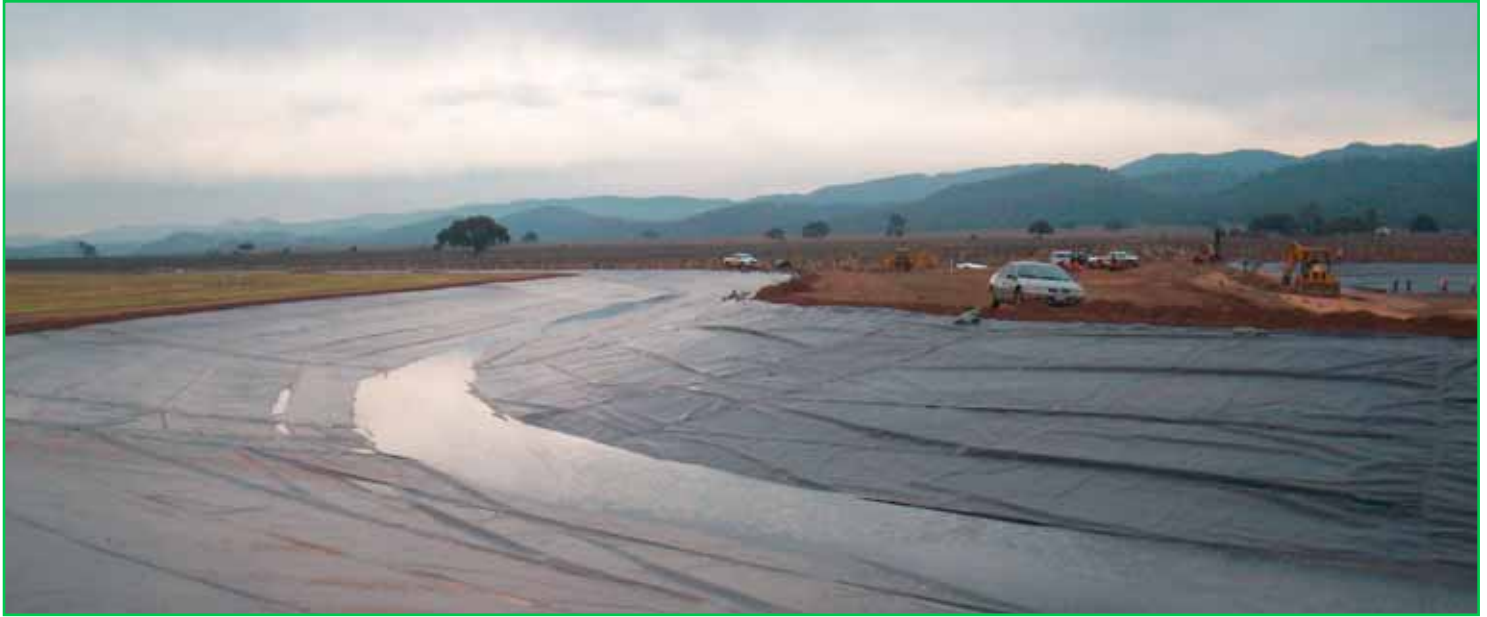
Canal lined with factory fabricated geomembrane.
