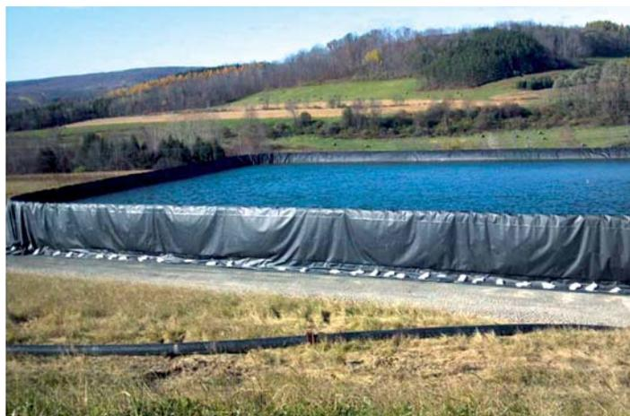
**FIGURE 2** Above ground drill pad water containment pond lined with a fabricated geomembrane.
