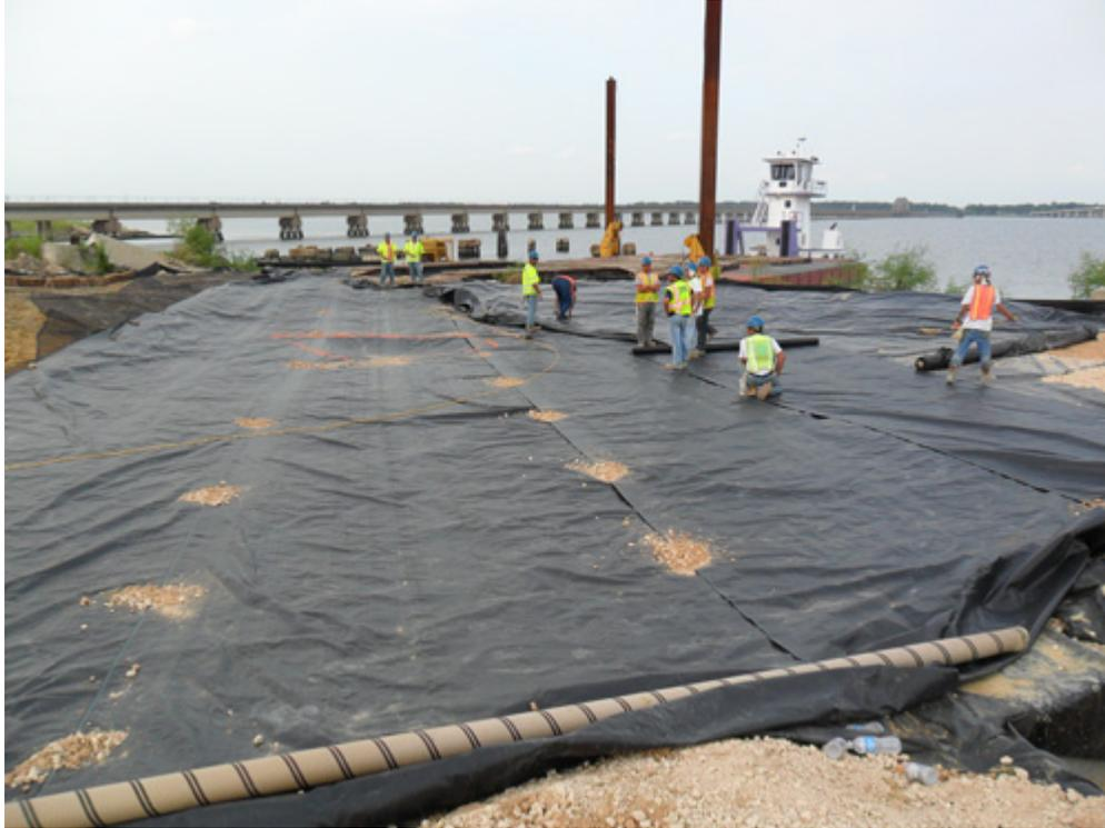
Engineered Textile Products built a decontamination station in Biloxi, Mississippi, using 30-mil reinforced geomembrane.
