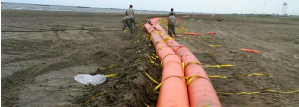
U.S. Flood Control installed 10 miles of Tiger Dams along the shores of Grand Isle beach in Louisiana, using Seaman Corporation's 28 ounce reinforced PVC geomembrane.
