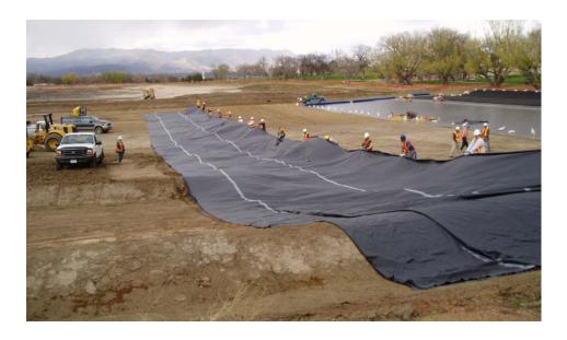
Flexible geomembranes are fabricated into panels in a controlled factory environment more suitable to high quality seaming than variable field environments. The size of panels is usually limited only by allowable shipping and handling weight. It is common to ship panels that weigh 1,816 kg (4,000 lbs) but panels as heavy as 4,086 kg (9,000 lbs.) have been shipped. On-site,
