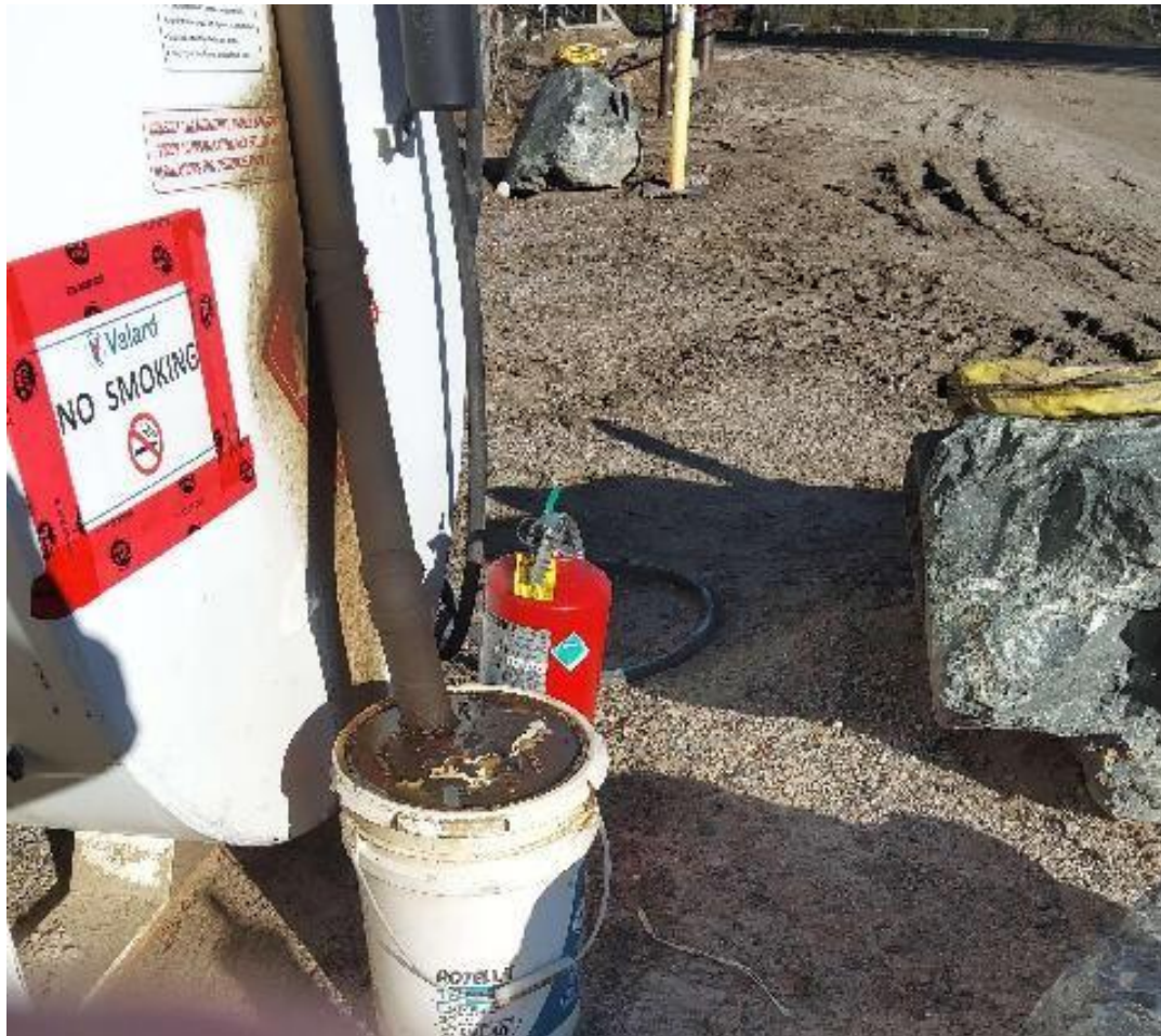
Figure 1: Drip bucket for fuel nozzle is full of water and fuel
