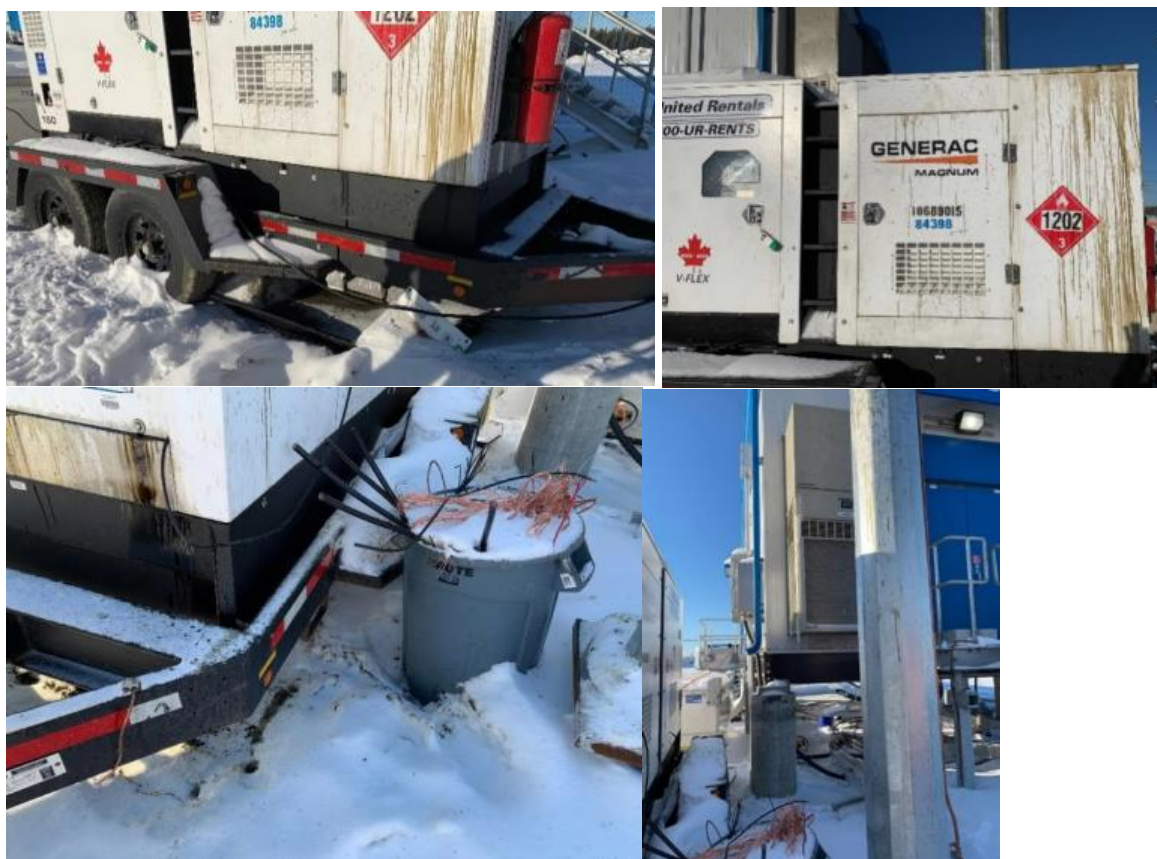
Photo 14: Substation C – Diesel sprayed from generator. Covering the surrounding area (snow, building, pole). Clean-up required.
