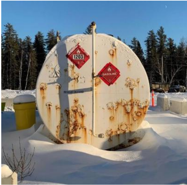
Photo 7: Pickle Lake Camp, Material Yard and Substation B – Gas tank by the Pickle Lake office, showing signs of corrosion/rust. Spoke with Katey and she confirmed it is only superficial. Need inspection logs to verify.
