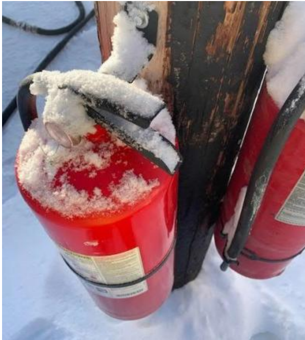
Photo 1: Sioux Lookout Camp and yard – Extinguisher by fuel tank does not have an inspection log.
