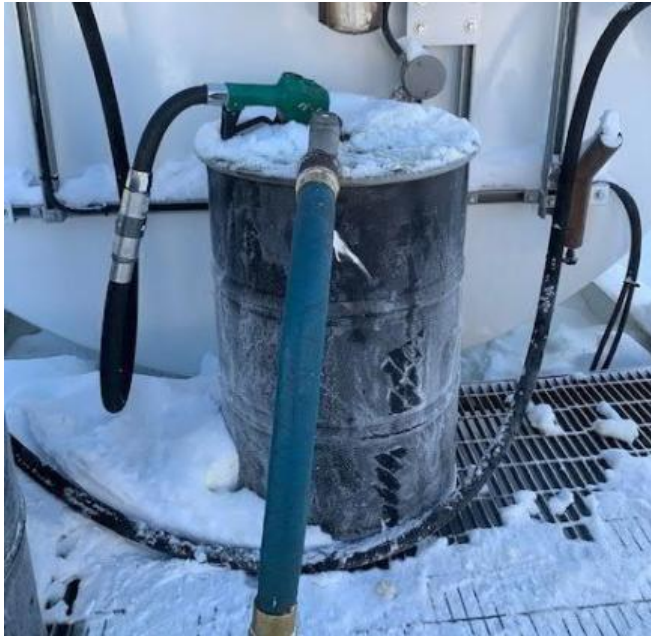
Photo 4: Sioux Lookout Camp and yard – Gas nozzles left in can, not in the holster.
