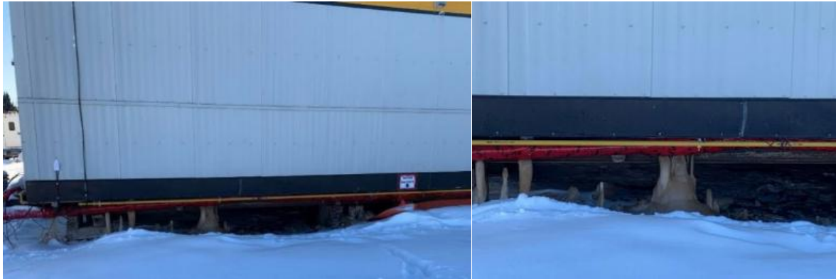
Photo 11: Pipestone Camp – Leaking pipe under rec trailer.
