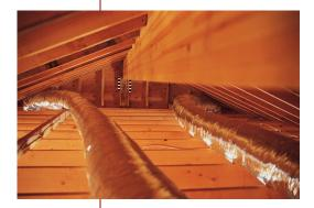
Duct work is installed as needed in attics, ceilings and walls to distribute heated air in the winter and cooled air in the summer.
