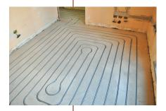
Tubing installed in the slab (for basement) or under a layer of gypcrete is connected to manifolds that pump warm water through the system.
